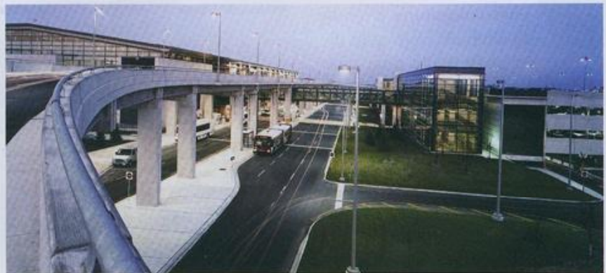
▲ Many security systems are brought together in airport security solutions. (Photo courtesy of Pelco)
